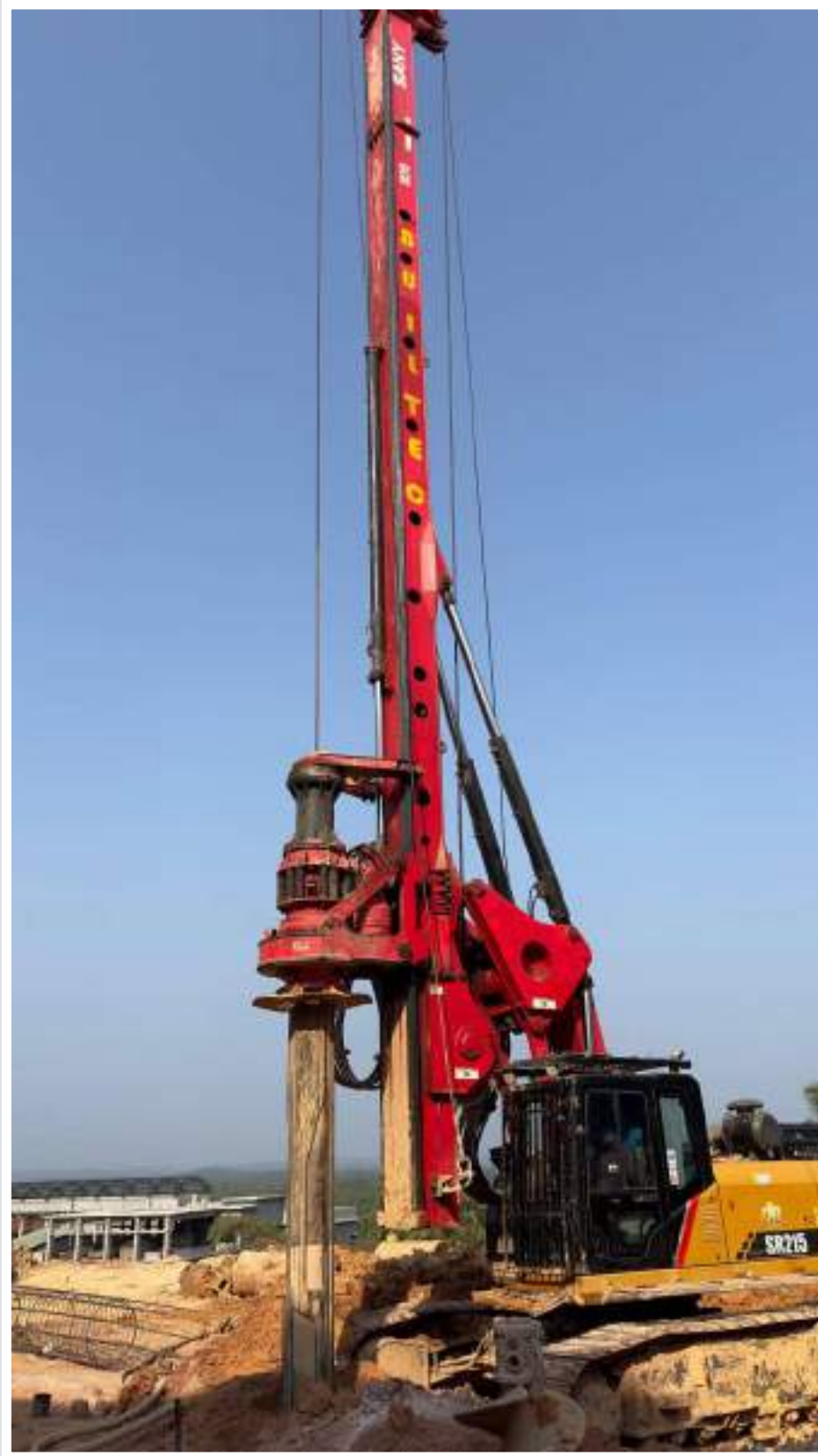
Advanced rig equipment for piling work
