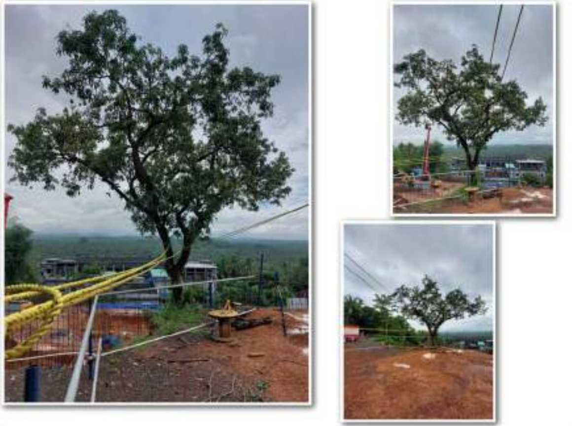
Preservation of existing trees during excavation
