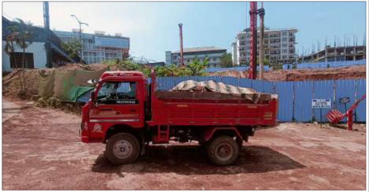
Using appropriate methods to prevent dust during soil shifting
