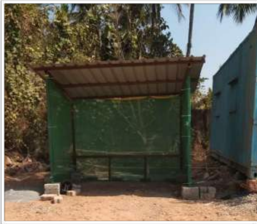
Shelter for laborers to rest at site
